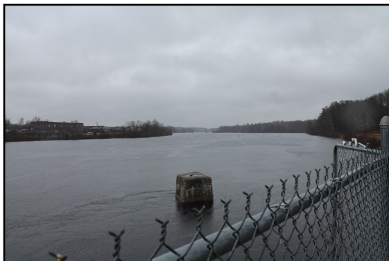
View upriver from Waterville Dam.
