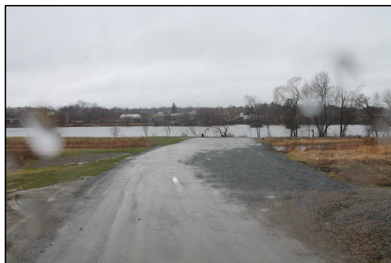
Access road to Kennebec/Messalonskee Trails parking area north of the Waterville Dam.
